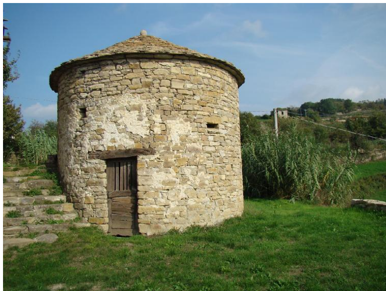
Figure 16: “Scau” Chestnut Drying Structure
